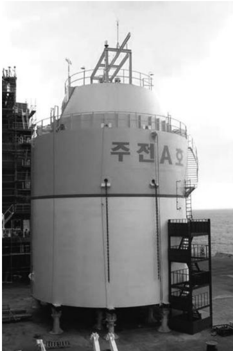
FIGURE 13.4 (See color insert.) CHUJEON-A, a prototype of wave power. (From Jeon, B.-H. et al., Autonomous control system of an induction generator for wave energy device, Ocean Development System Lab., Korea Research Institute of Ships and Ocean Engineering, KORDI, Daejeon, Korea, Proceedings of The Fifth ISOPE Pacific/Asia Offshore Mechanics Symposium , Daejeon, Korea, November 2002, pp. 17–20.)
