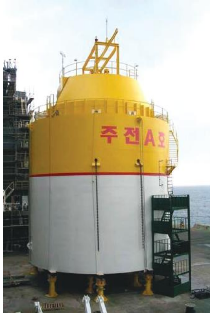
FIGURE 13.4 CHUJEON-A, a prototype of wave power. (From Jeon, B.-H. et al., Autonomous control system of an induction generator for wave energy device, Ocean Development System Lab., Korea Research Institute of Ships and Ocean Engineering, KORDI, Daejeon, Korea, Proceedings of The Fifth ISOPE Pacific/Asia Offshore Mechanics Symposium , Daejeon, Korea, November 2002, pp. 17–20.)
