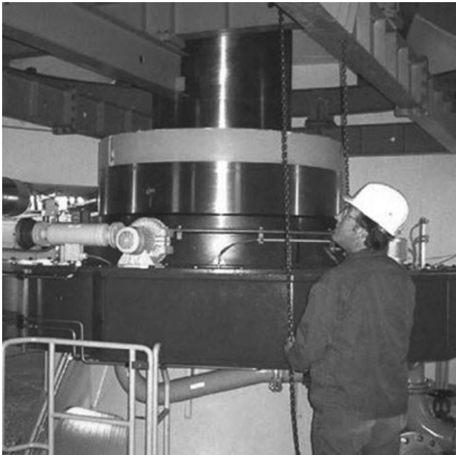
FIGURE 13.9 (See color insert.) Shaft between the induction machine and the turbine.
